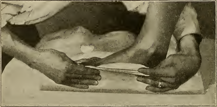
CHART No. 218 Heaping Plaster Under the Arch.
